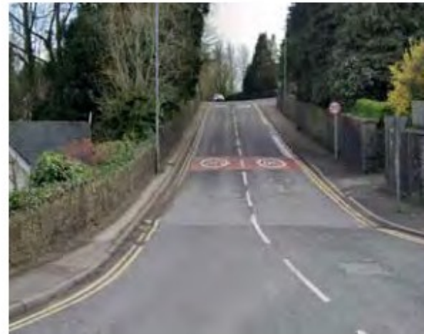
Narrow footways on busy road
