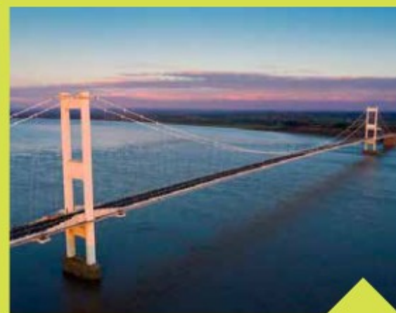
M48 Severn Bridge
